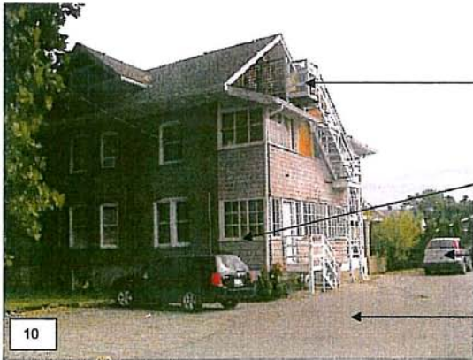
South elevation of building.
