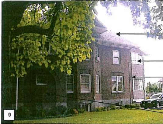
West elevation of building.
